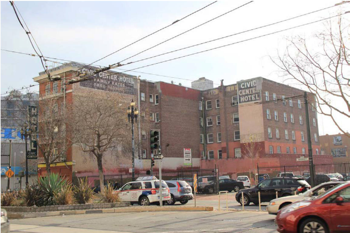
Interior - (west-) facing facades
