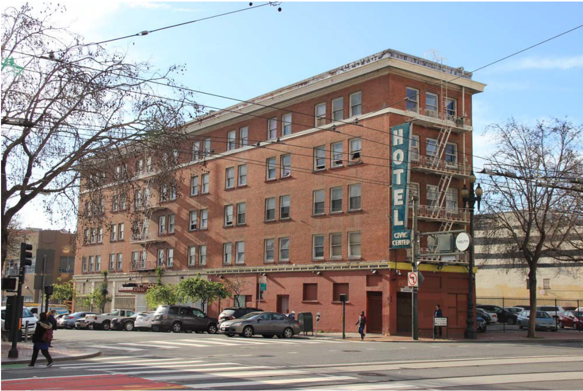
Primary (12th Street) Façade and secondary (Market Street) facade, looking south from across Market Street
