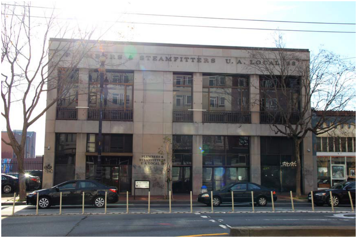
Primary (Market Street) facade
